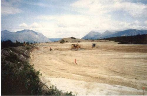
Photo 1 – Existing tailings impoundment being regraded by a D8 and D4 dozer, July 1999.
